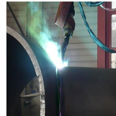
welding of filling/cap passes
