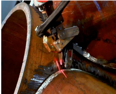
Measurement of seam preparation with laser scanner
